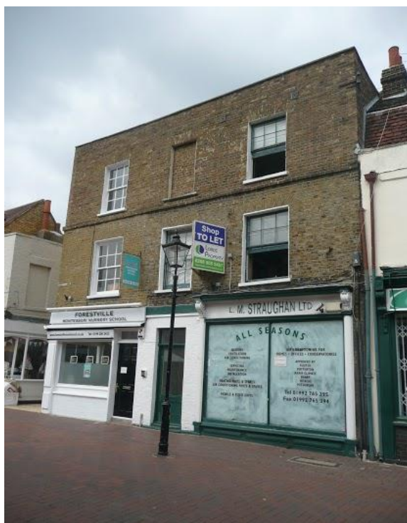
Vacant shops, Sun Street (EFDC)
