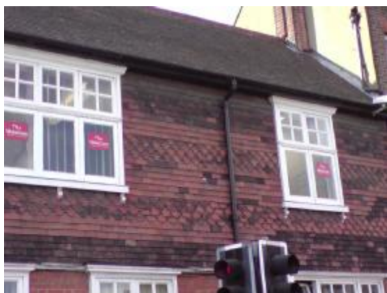
Hanging tiles (EFDC)
