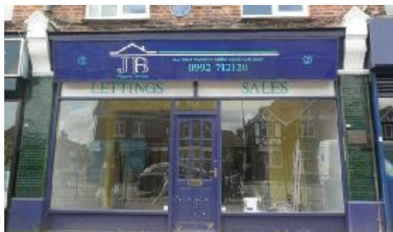
Tiled pilaster with decorative console (EFDC)
