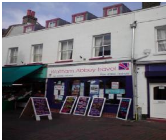
Large adverts and excessive signage (EFDC)
