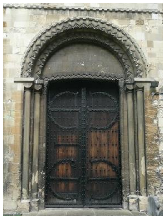
Norman south door featuring a pair of substantial timber doors with large iron strap hinges set in a Norman arch, Abbey Church (EFDC)
