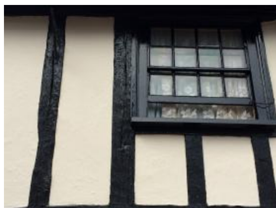
Traditional timber framing (EFDC)
