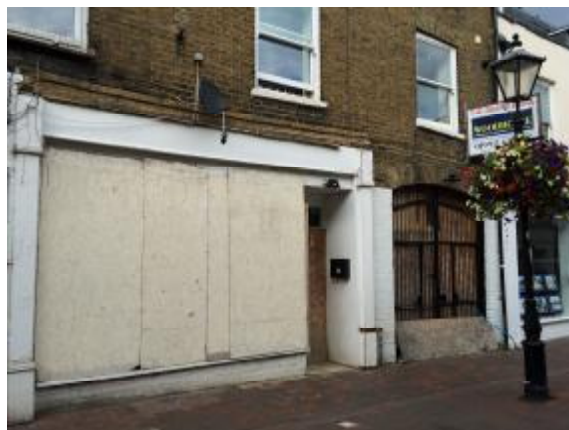
Vacant shops, Sun Street (EFDC)
